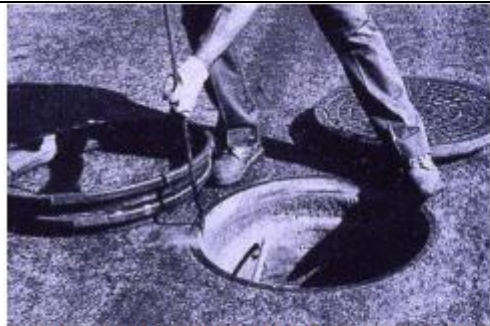
a. Clean Up Existing Manhole Ring & Cover
