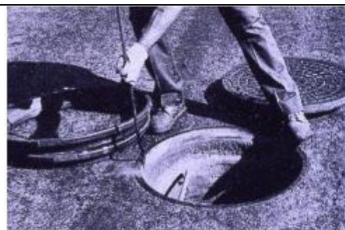
a. Clean Up Existing Manhole Ring & Cover
