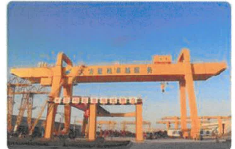
300t Double Girder Test Platform
